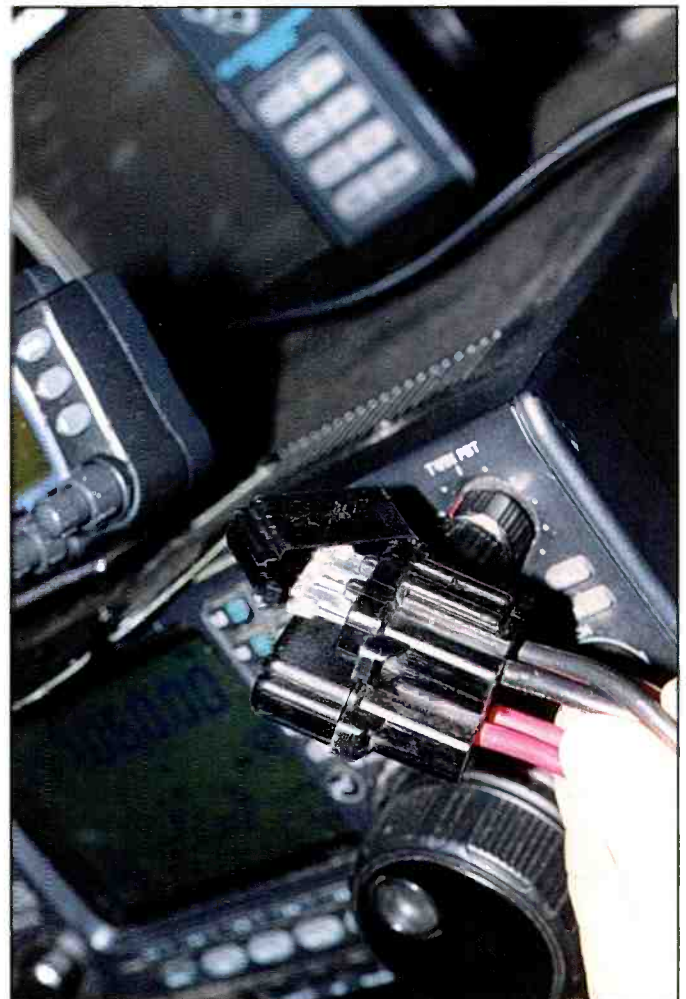
Surprise! The black fuse was blown.
