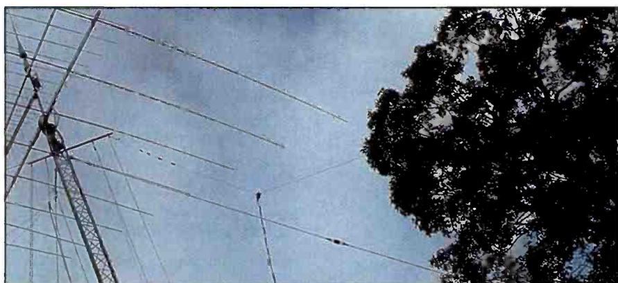
Photo B. My Eavesdropper was installed as a sloper. The high end is supported by a 60-foot tower. If you look closely, you can make out the top four traps to the left of the tower (other wire antennas, guy wires, and clutter precluded getting a clearer shot of the installation).
